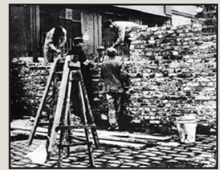
Warsaw Ghetto wall being built, 1940.
