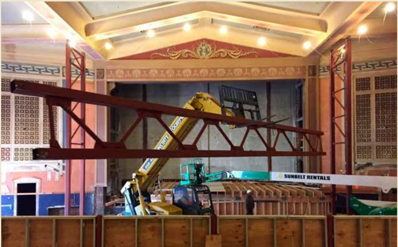
Raising the truss. Photo: David Mayeri
