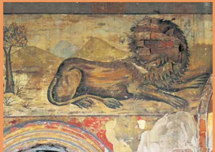
Synagogue wall, pre-renovation, Dąbrowa Tarnowska. Photo by Chris Schwarz
