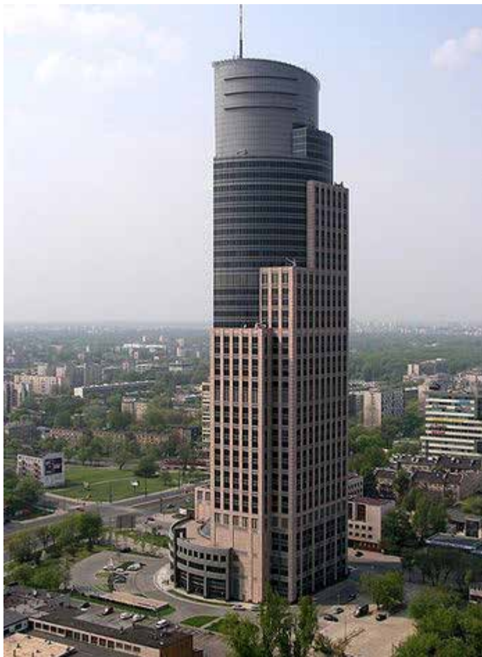
The Warsaw Trade Tower, the fourth-tallest building in Poland and Poland's largest office building, purchased by Mitzner's Apollo-RIDA development corporation
