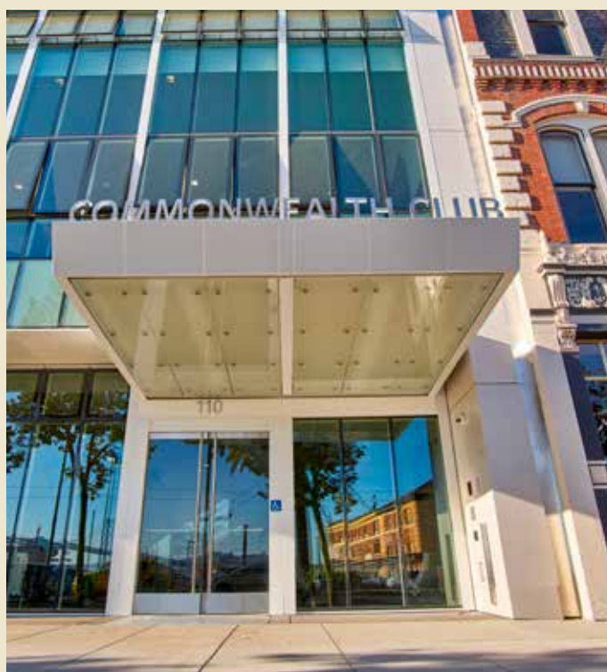
New home of Commonwealth Club of California
